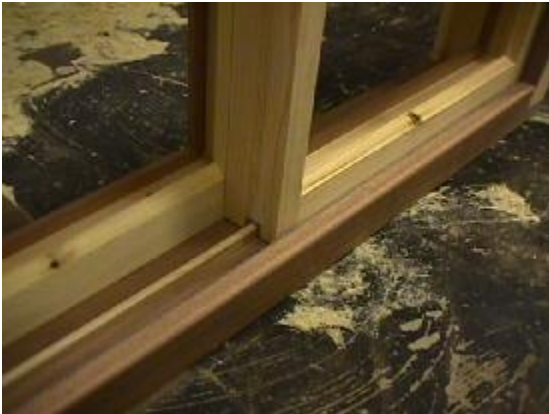
Opening sash showing guide rail and plough in sash
